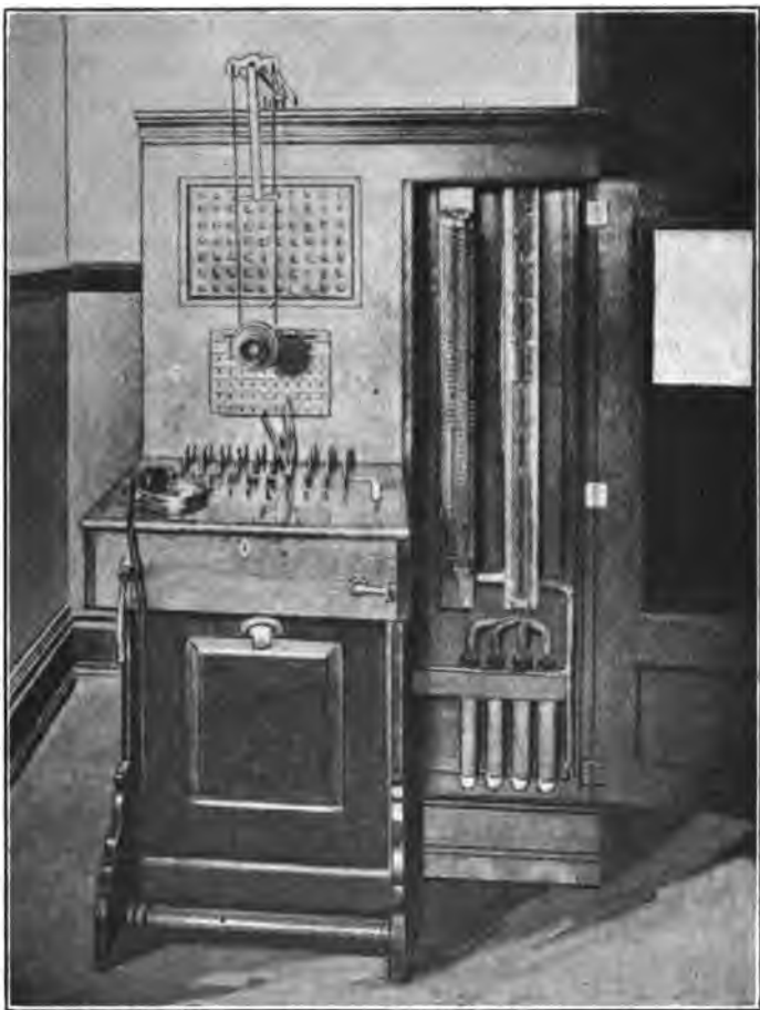
FIG. 107.—Switchboard installation (terminal cabinet on right).
